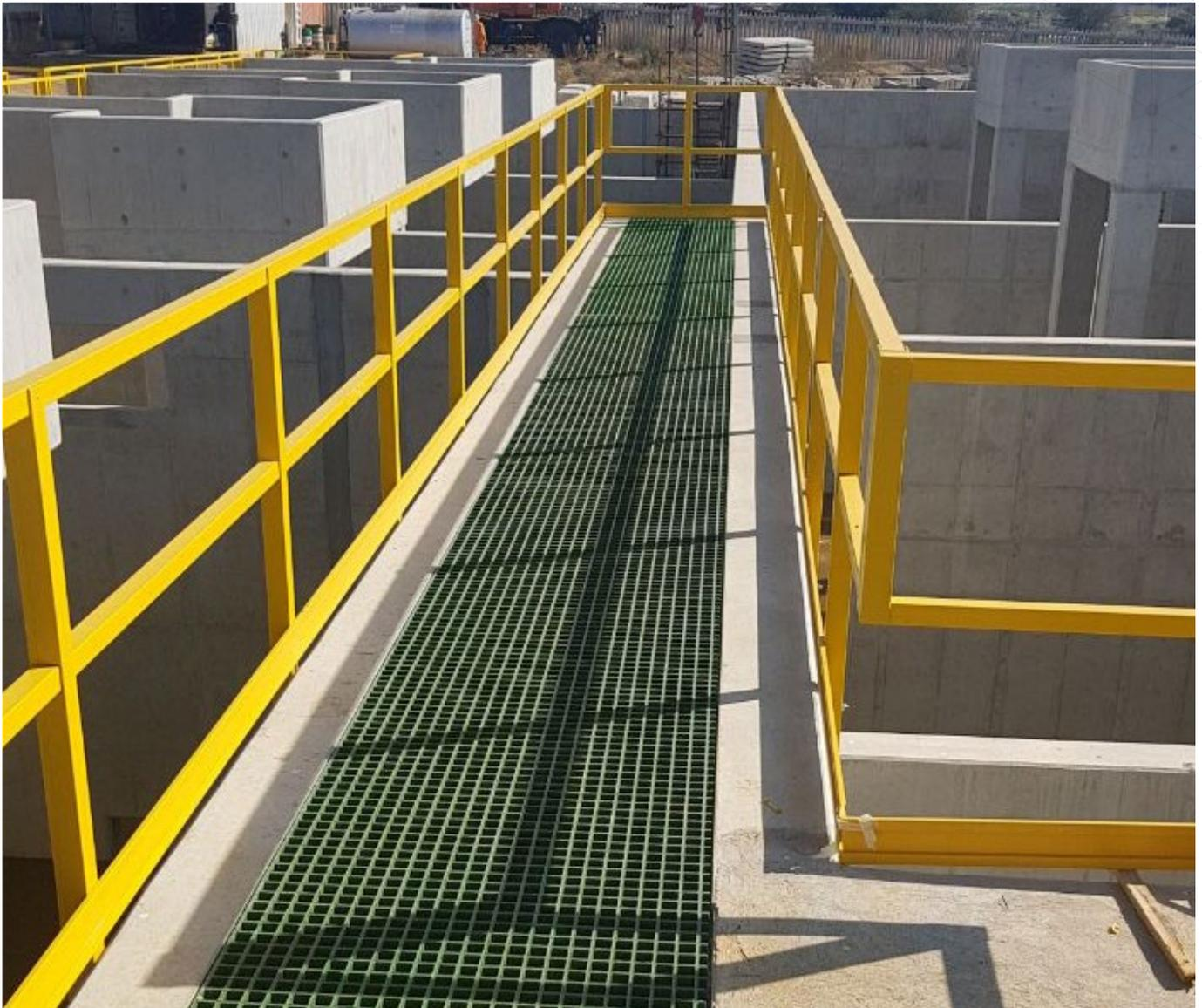
38mm GRP Grating and 44mm Square Tube Hand Railing
